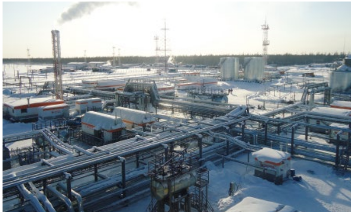
▲ Taas-Yuryakh central processing facility at the Srednebotuobinskoye oil and gas field during the Siberian winter.
