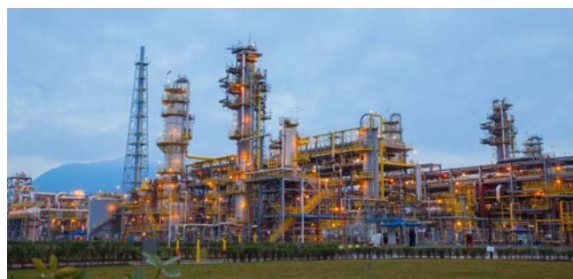
Photo: First production from the Chuandongbei natural gas project in the Sichuan Basin was achieved in January 2016.
