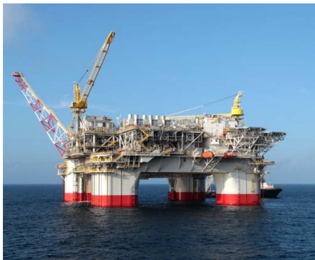
Photo: Production ramp-up continued at the Jack/St. Malo semi-submersible floating production unit.
