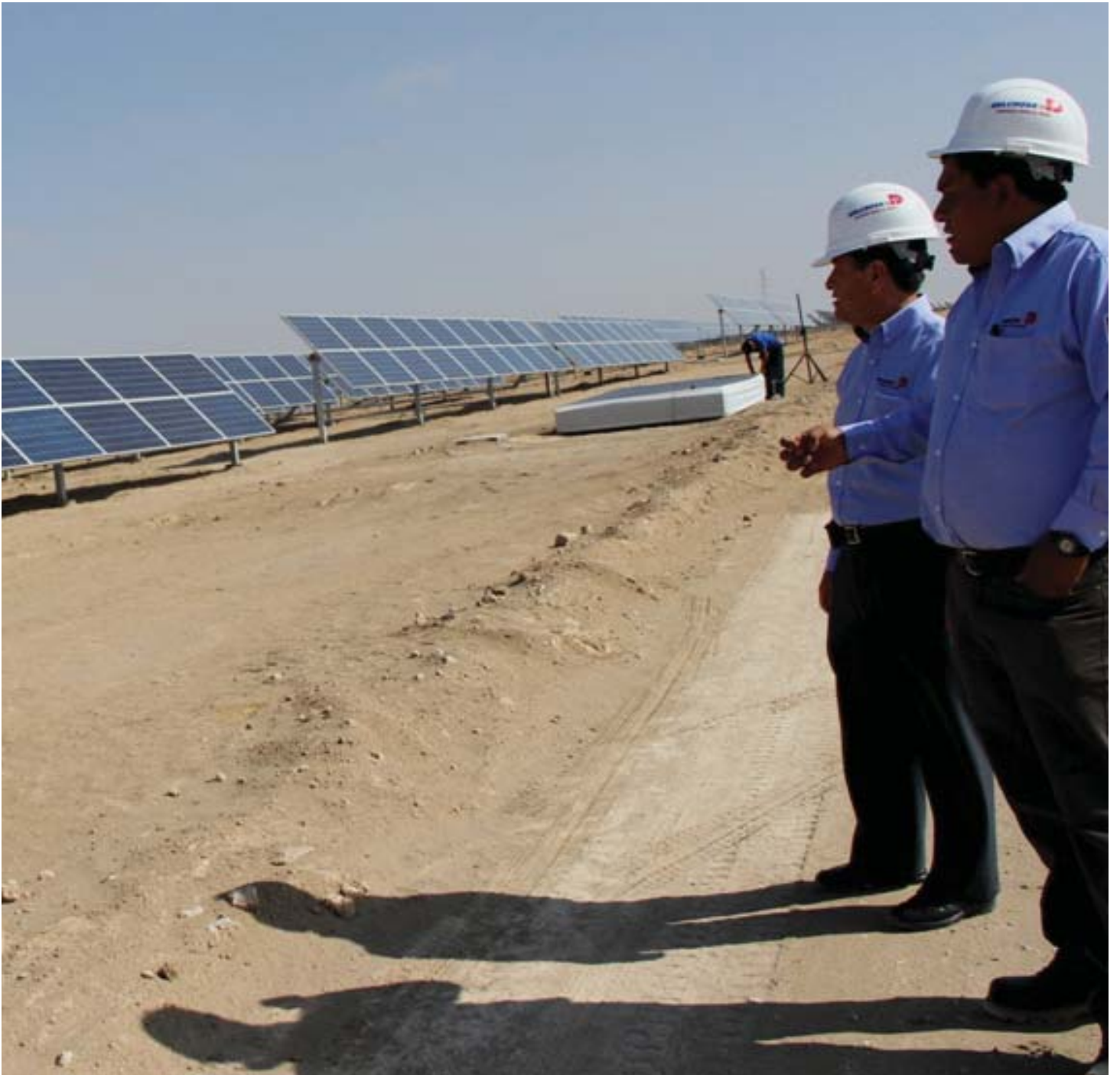
Solar PV Plant in Peru Photo Courtesy: MINEM Peru
