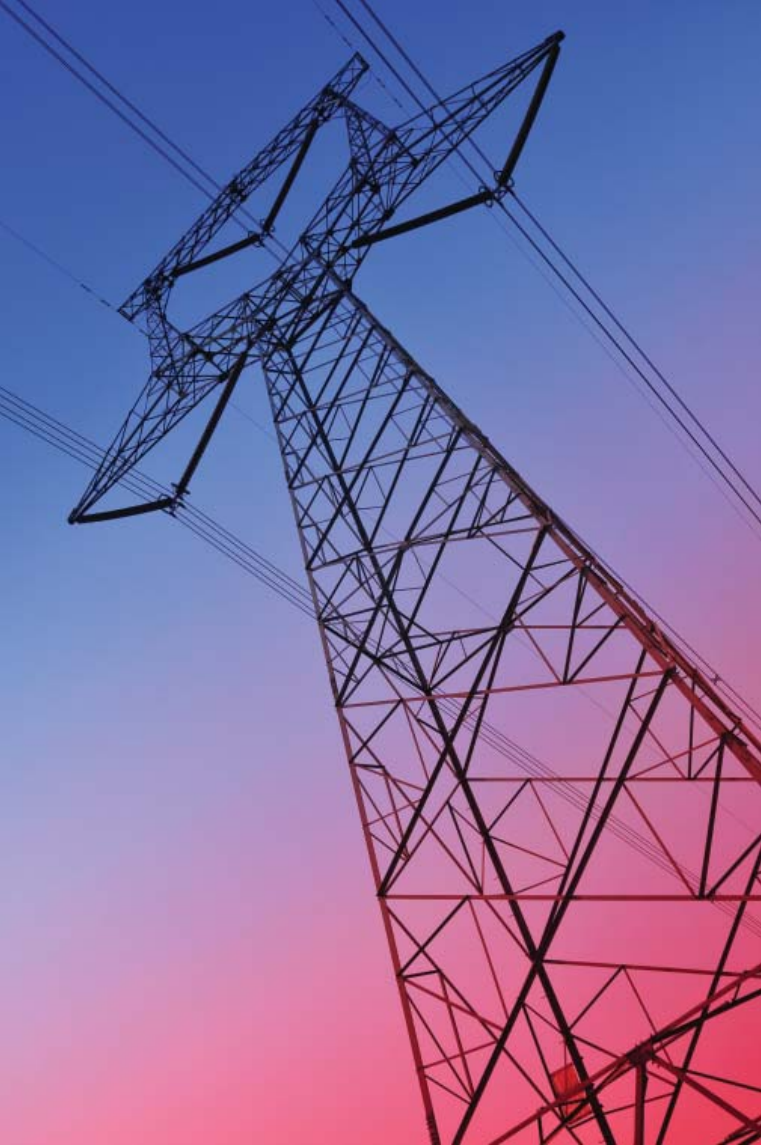
Transmission tower Photo Courtesy: Shutterstock
