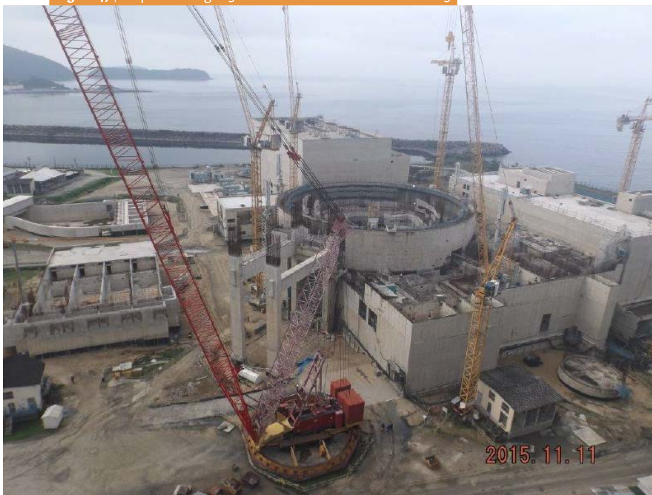
Figure 47 | Suspended Angra-3 Construction Site in November 2015
