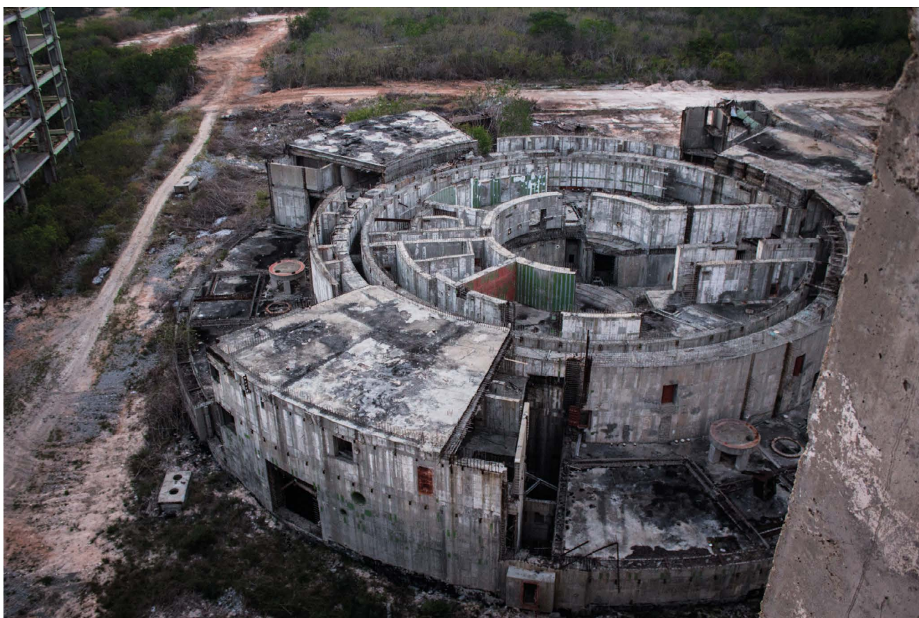
Juragua site in Cuba, where building of two Russian-designed 413 MWe reactors started in 1983 and was abandoned in 1992. Photography by © Darmon Richter, August 2014, see http://www.thebohemianblog.com/2014/08/cuba-abandoned-unfinished-soviet-nuclear-power-station.html .
