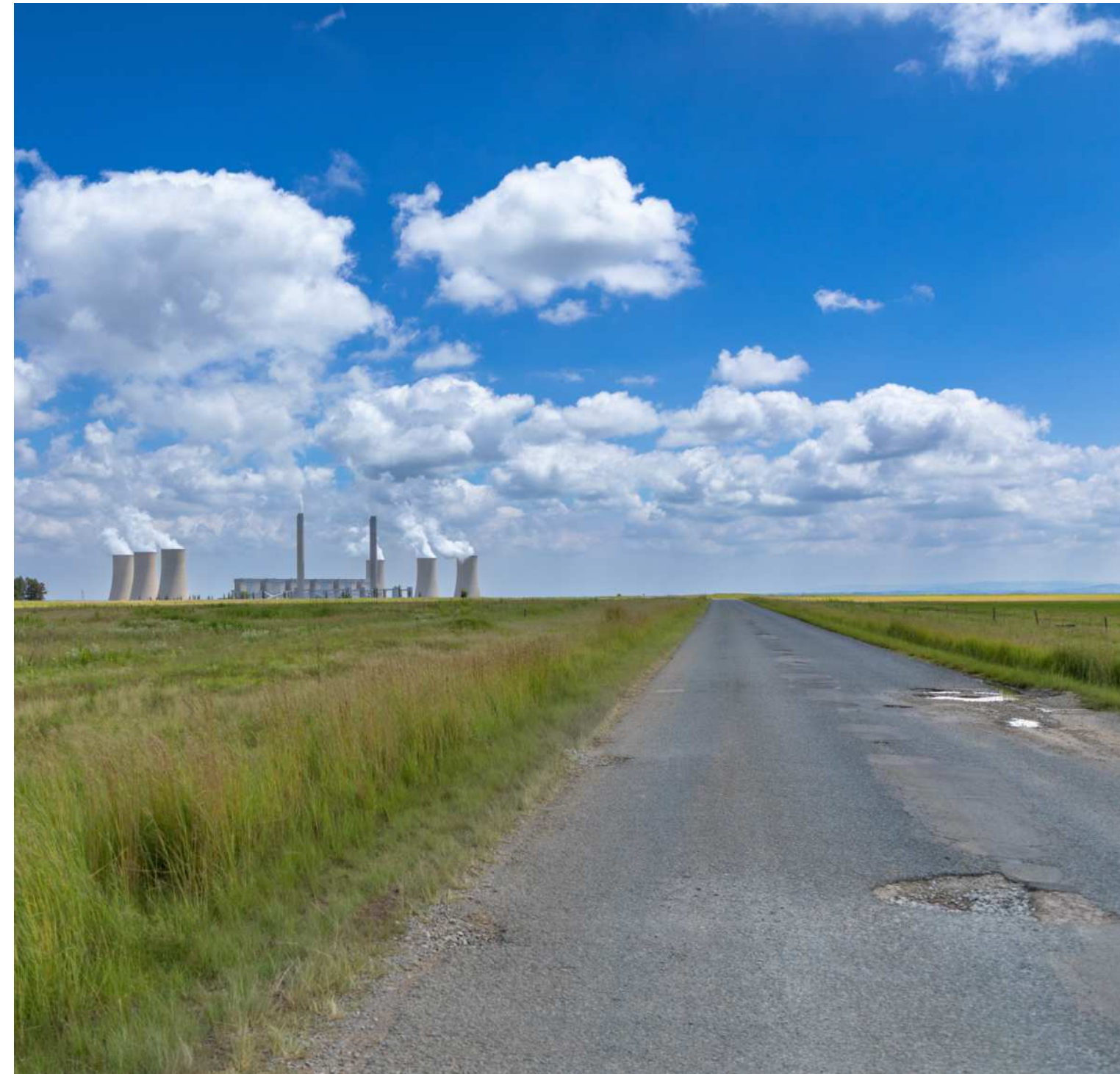
One of 13 coal-fired power plants in South Africa owned and operated by the country's highly indebted utility, Eskom. A rapid, large-scale renewable energy build-out is vital in South Africa to replace the ageing and poorly maintained fleet of coal plants. A lack of generation capacity caused by persistent breakdowns has led to thousands of hours of load shedding in 2022 alone, causing significant hardship and damaging an already-challenged economy.
