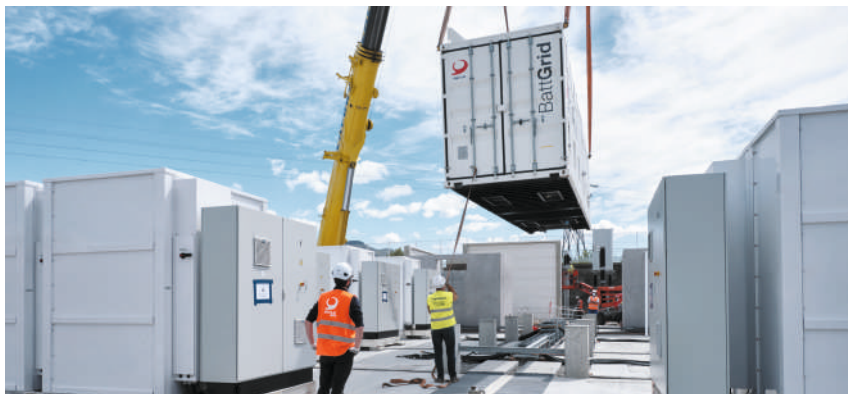
Installation de batteries
